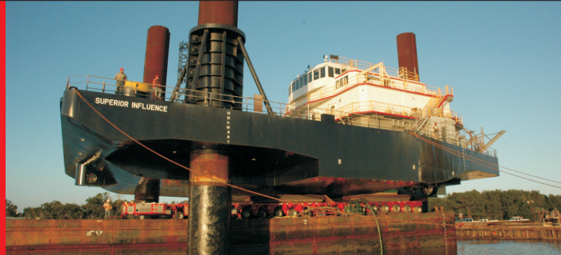
The vessel beginning its ascent from the transporters & barge.
